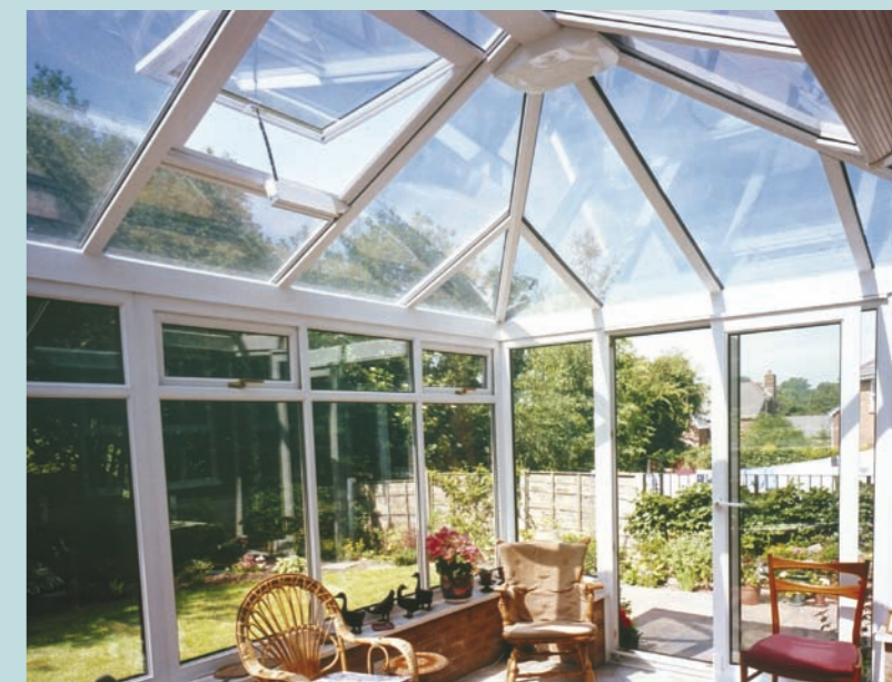
Thermally efficient glass roof
